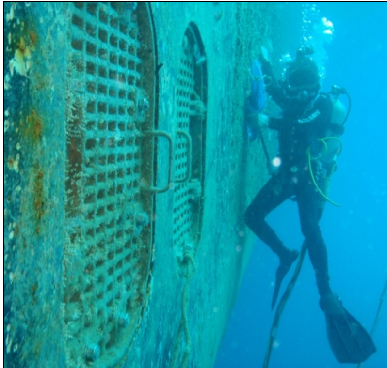
Figure 6 A diver conducting an in-water inspection of an oil rig pontoon
