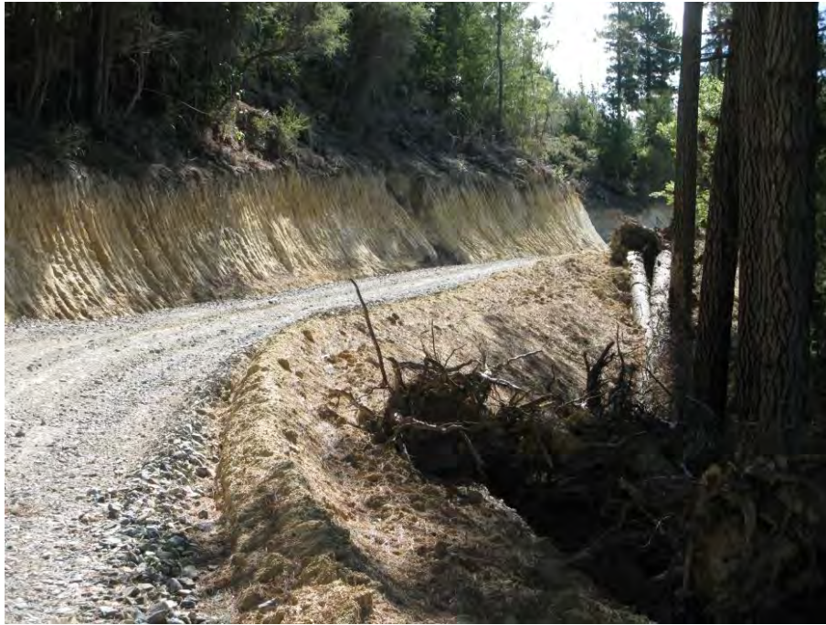
Figure 3: Road constructed on highly erodible Separation Point Granites (SPG). SPG are identified within the Plan as occurring within the Orange Zone, with afforestation as a permitted activity.
