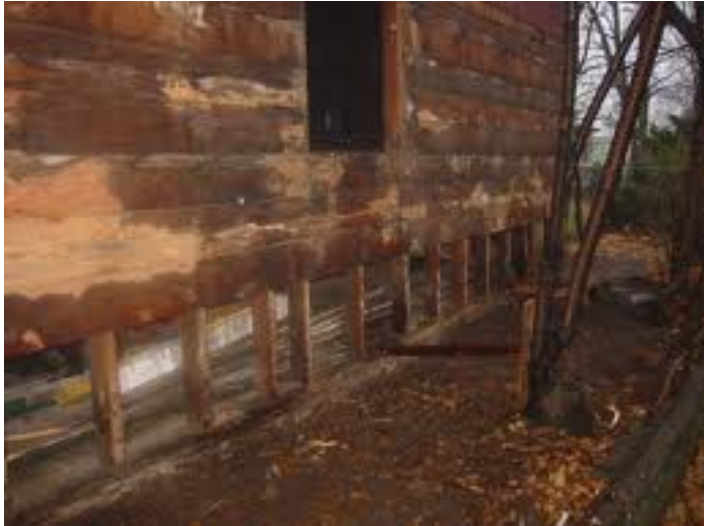
Effect of termite damage
