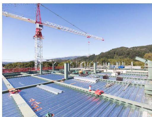
28 March 2017: Contractors begin installing the floor on the upper level of the building, getting ready to pour concrete
