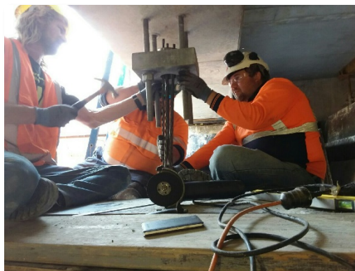
Contractors connect the anchor piles to the underside of the new lab
