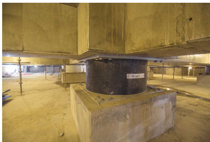
The lead rubber bearings are in the basement, sitting above the underground foundations.
