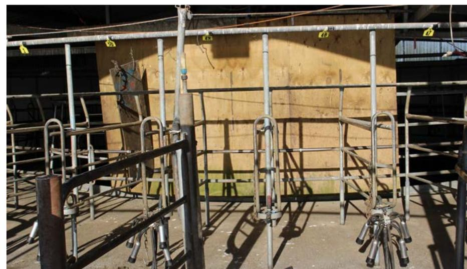
Panels have been erected directly in-line with the cow entry to the milking platform, which prevents the cows being unsettled by herd testing equipment and other work undertaken within the centre of the turntable.
