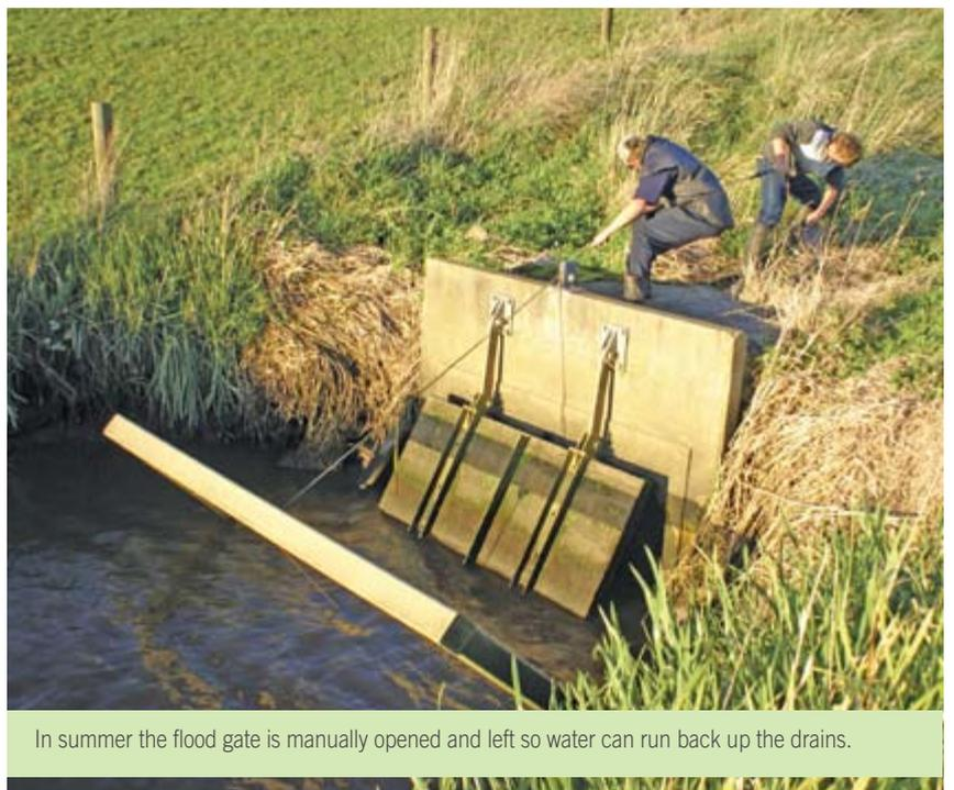
In summer the flood gate is manually opened and left so water can run back up the drains.
