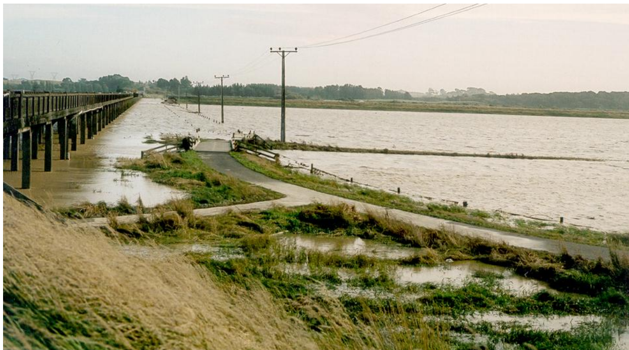
Extensive flooding at Foxton
