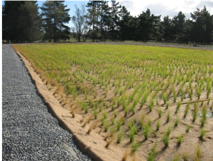
Figure 5: Example of a floating wetland designed for nutrient removal from a municipal/industrial wastewater treatment pond (with permission from Waterclean Technologies, NZ).
