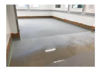
Following this the first MMA membrane is poured out on the level floor - this is a self-levelling liquid product, approximately 1.5mm thick. Next, a wearing layer is poured, this is slightly thicker at 2mm and now things have to move quickly as the multi-coloured fleck finish must be applied before it dries. Workers hand cast the fleck, so applying a consistent spread requires a practised technique. After curing, any excess fleck is collected up to be used again.
