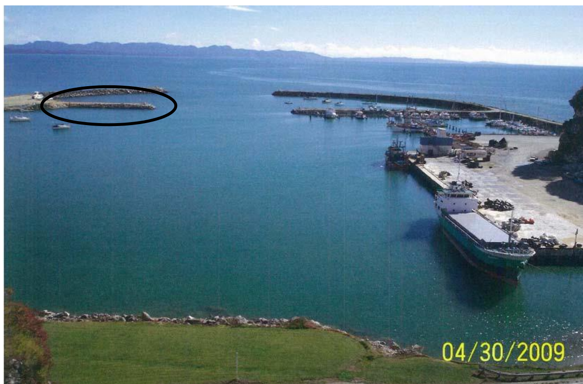
Figure 21: Port Taranaki illustrating a recent extension of the western breakwater (circled) (after Tasman District Council 2009).
