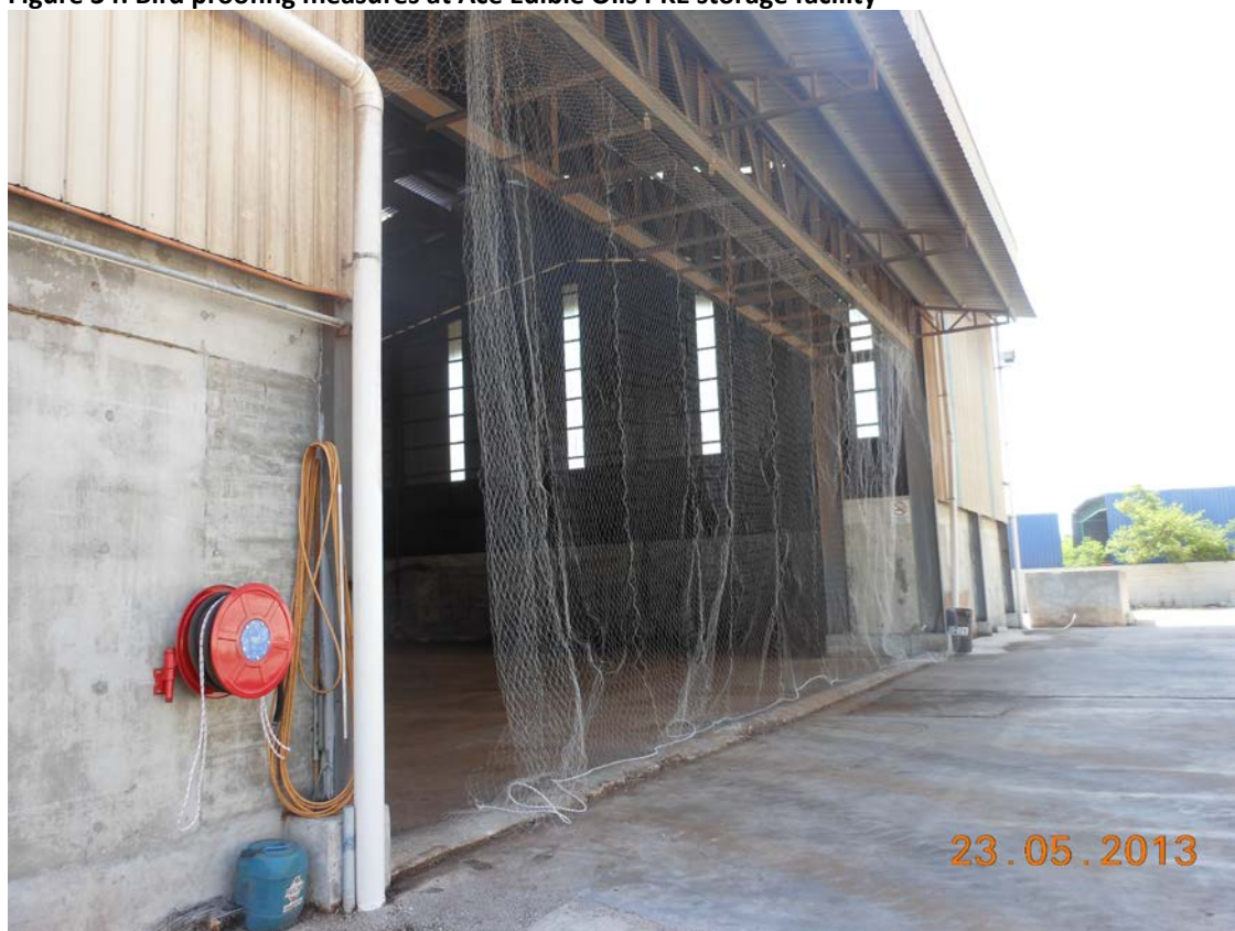
Figure 34: Bird proofing measures at Ace Edible Oils PKE storage facility
