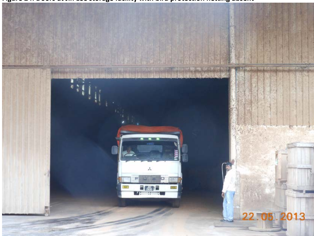
Figure 24: Doors at Jin Lee storage facility with bird protection netting absent
