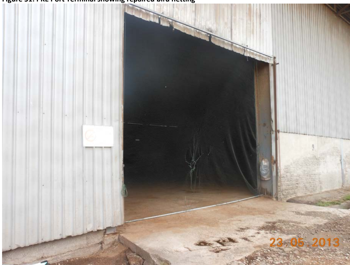
Figure 51: PKE Port Terminal showing repaired bird netting
