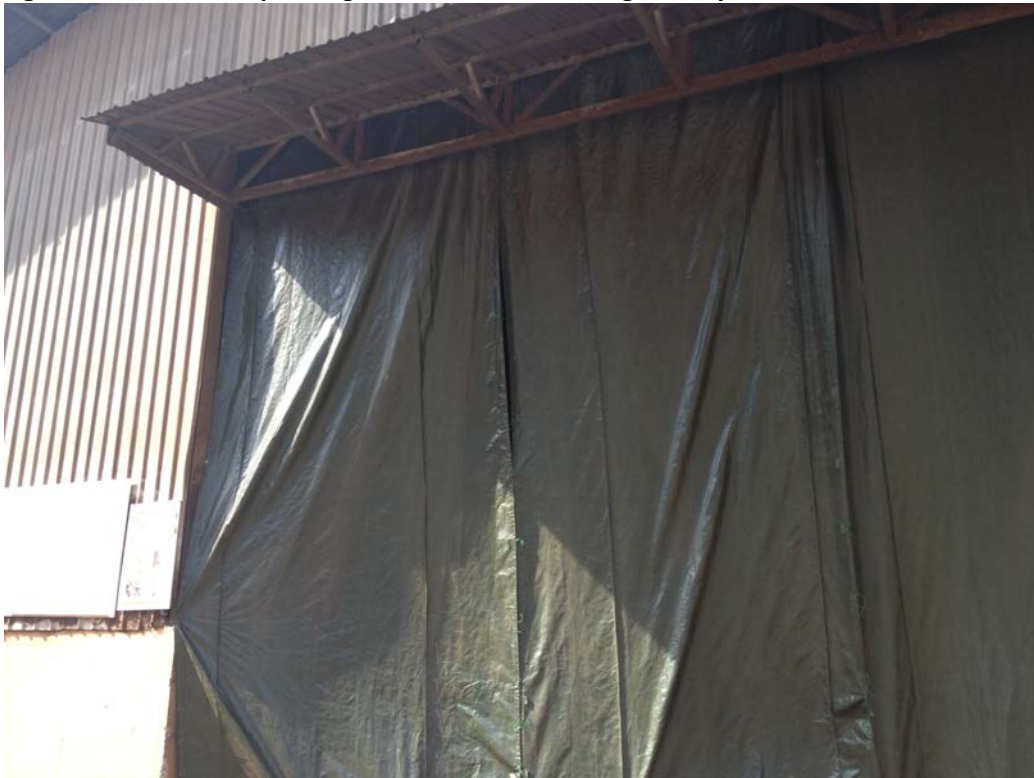
Figure 5: Photo of Bird-proofing sheets at doors of storage facility
