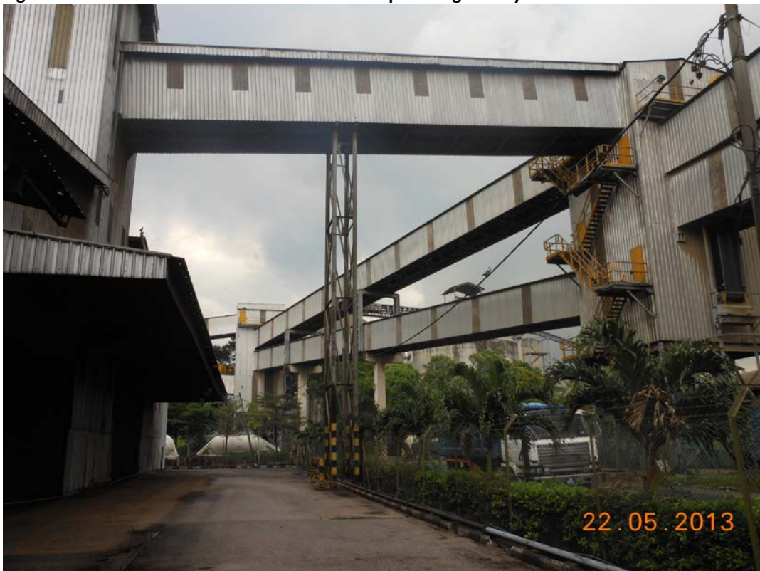
Figure 47: PKE Jahor Port Warehouse covered ship loading conveyors
