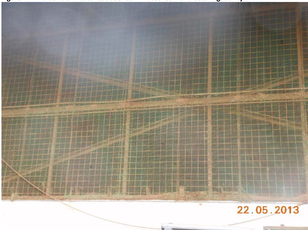
Figure 27: Bird control measures at Sehcom Industries manufacturing facility
