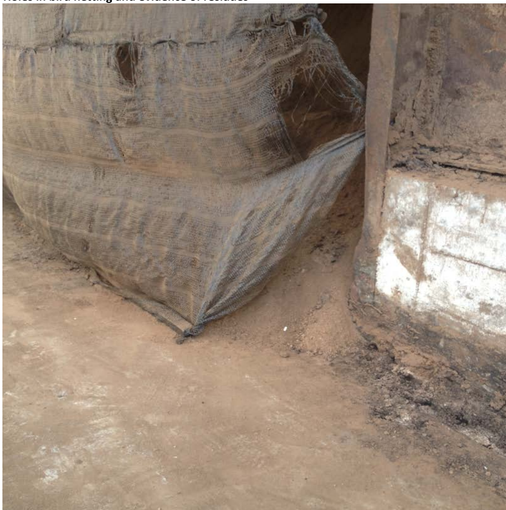
Figure 39: Holes in bird netting and evidence of residues
