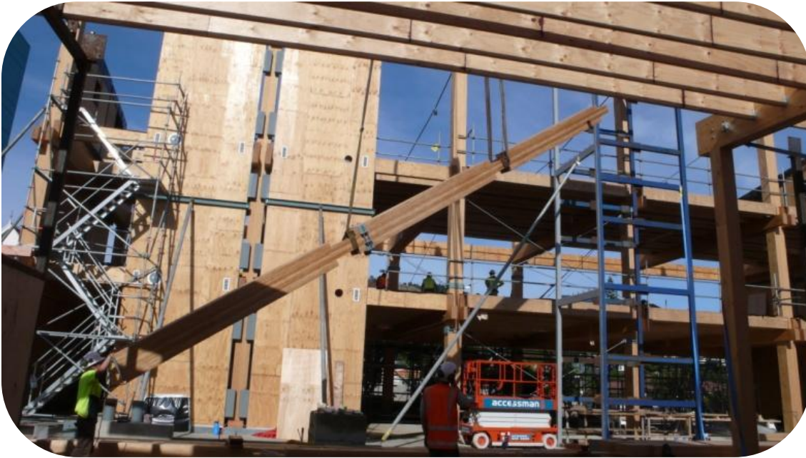
Figure E.20 Structure taking shape, shear walls in position and final columns being lifted into position. The Workshop structure is in the foreground.
