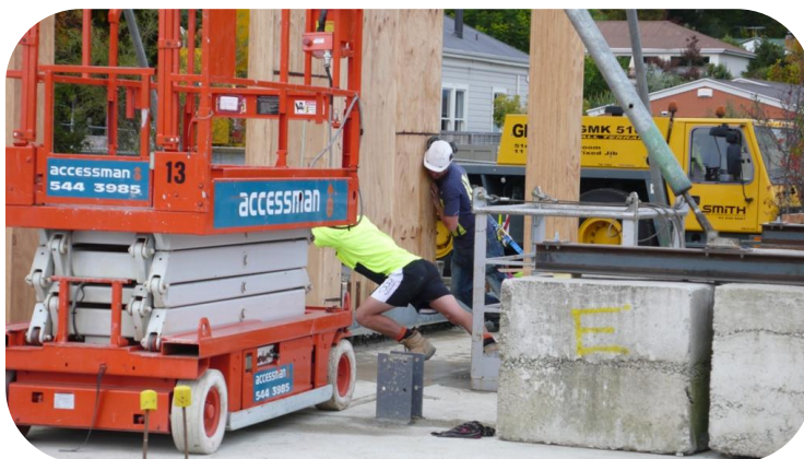
Figure E.12 Manoeuvring the base of the shear wall into the steel shoe.
