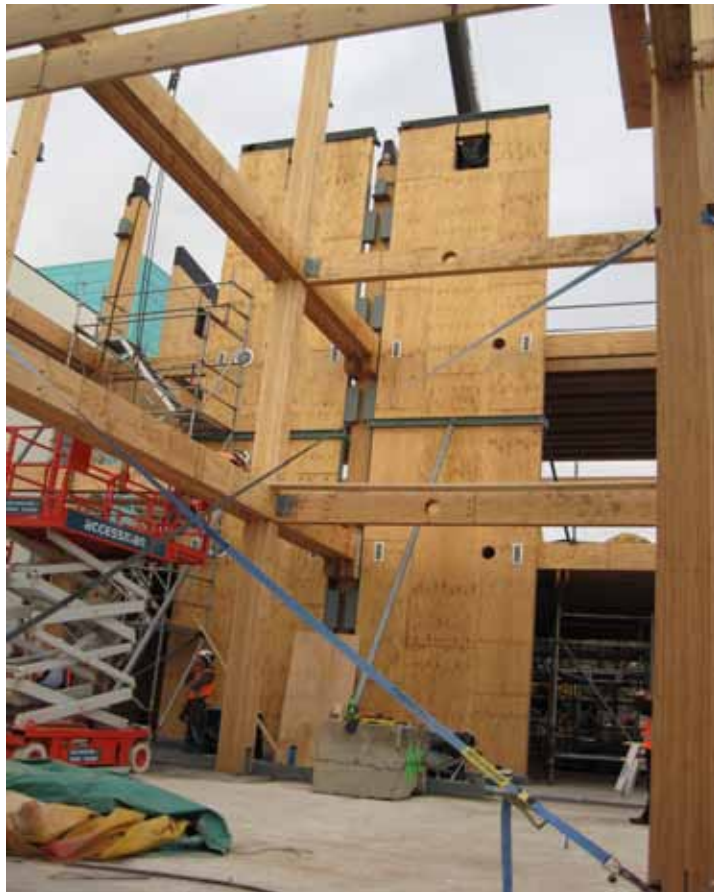
The massive timber (LVL) shear-walls of the Arts and Media building. (Photo by David Carradine)
