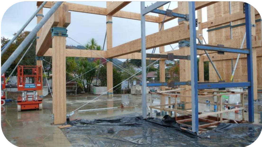
Figure E.16 Interior temporary bracing to frame. The collars to attach the bracing have to be carefully fitted to ensure minimal marking of the timber surface.
