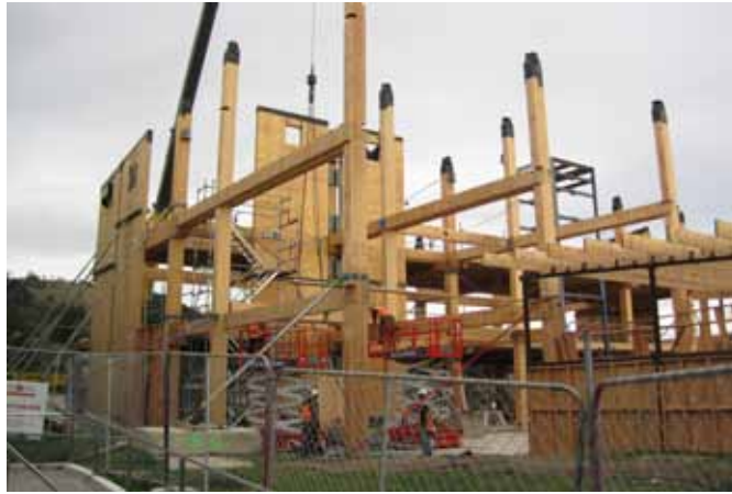
The structural timber (LVL) 'skeleton' of the Arts and Media building. (Photo by Andy Buchanan)
