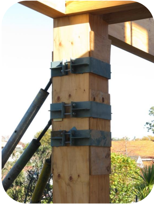
Figure E.29 Collars for temporary bracing to a column and protection to limit marking on timber surface.
