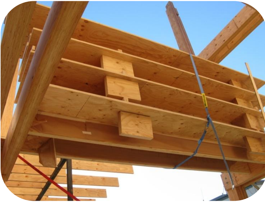
Figure E.22 Potius floor panels hoisted as a stack up to second floor level.
