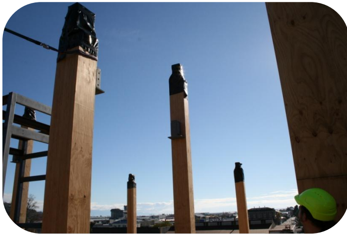
Figure E.30 Plastic covering on exposed end grain of columns to increase moisture protection over and above weather shield sealant.
