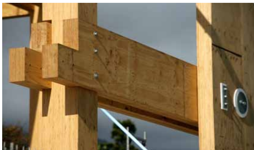
Detailing of beam / column joint on Arts and Media building. (Photo by Andy Buchanan)
