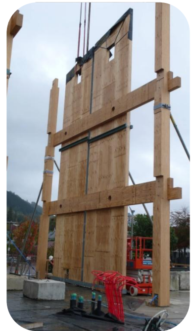
Figure E.11 Shear wall being placed into steel shoe.
