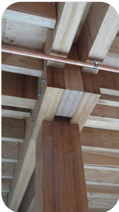
Figure E.38 Instrumentation to measure relative movement between LVL elements.
