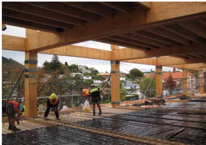
Preparing for pouring the concrete topping on top of the Potius floor units. (Photo by Andy Buchanan)
