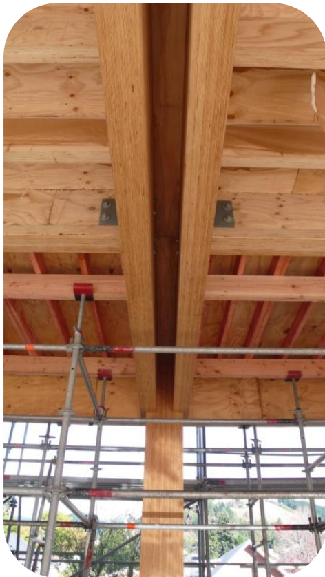
Figure E.27 Underside of second floor showing forming for cantilevered concrete section of floor to the south of the building.
