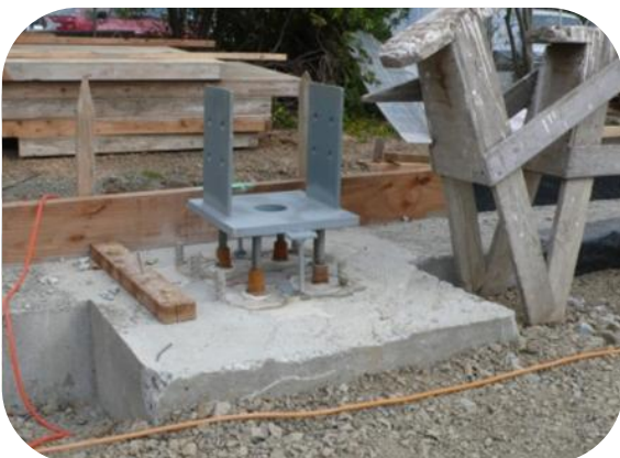
Figure E.6 Foundation and attachment for column. Note the elevation to allow floor slab to be poured.
