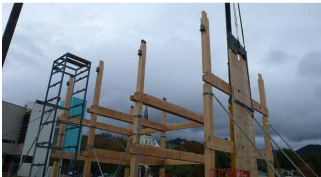
Figure 6.15: Protective weather capping on top of columns and walls.
