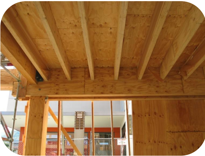
Figure E.26 Underside of second floor showing flanges of I floor panels.
