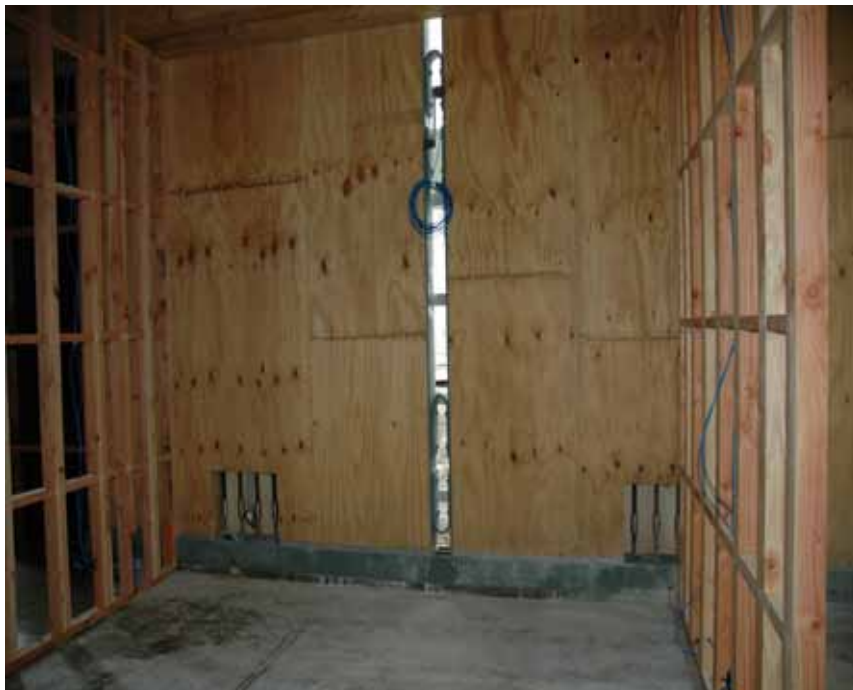
Paired shear-walls showing the Macalloy tensioning bars running vertically and the U-shaped energy dissipaters. (Photo by David Carradine)
