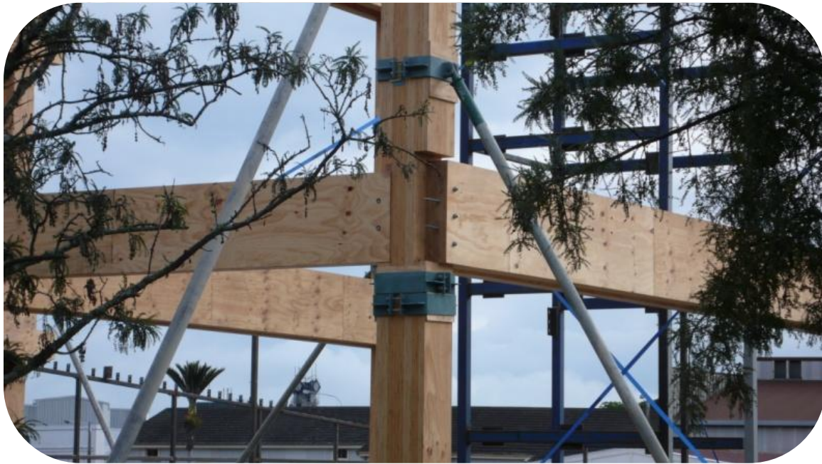
Figure E.13 Connection between column and beams. There is one more bay to be constructed to the right, the beam of which will be connected to the rods epoxied into the existing right side beam.
