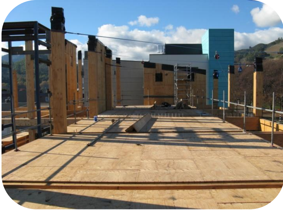
Figure E.32 Third floor level with Potius floor panels in place. View is looking along southern bay towards the east.
