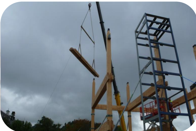
Figure E.9 LVL elements being moved around the site by crane. The increased height of the crane allowed elements to be lifted over the existing structure.
