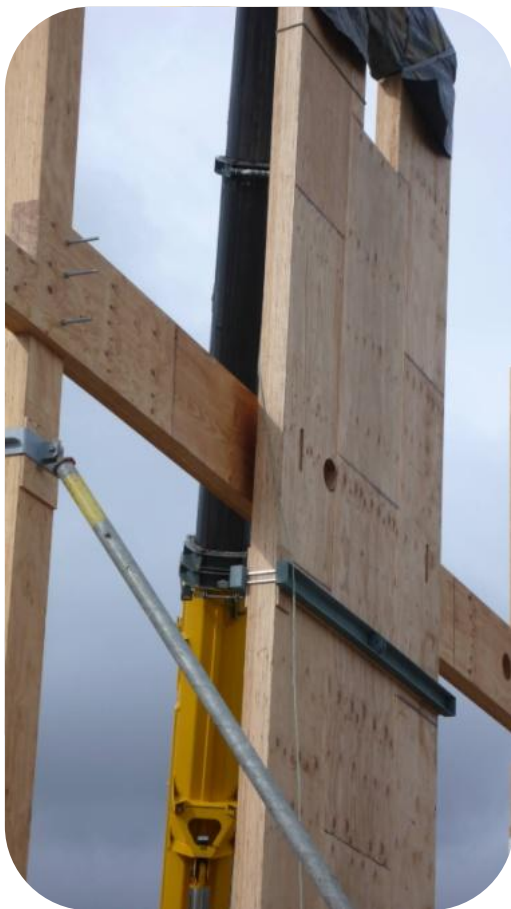
Figure E.14 Shear wall in position but not attached to corresponding beam.
