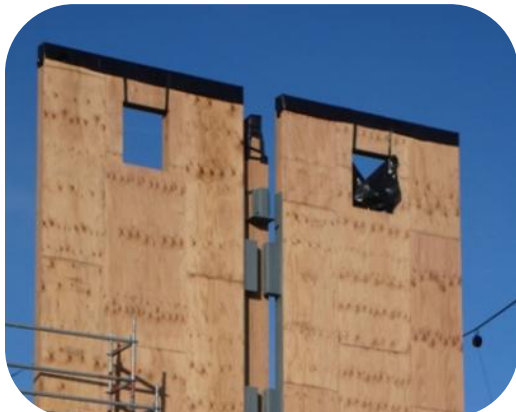
Figure E.31 Plastic capping to exposed ends of shear walls.
