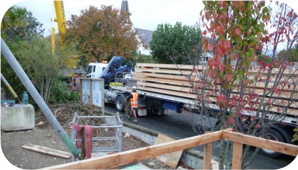
Figure E.7 LVL elements arriving at the site by truck. The elements are hoisted off the truck by crane – seen in background.
