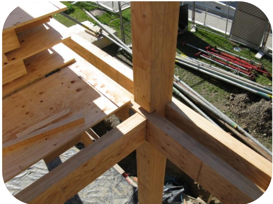
Figure E.23 Potius floor panels in position and others stacked ready to be placed.
