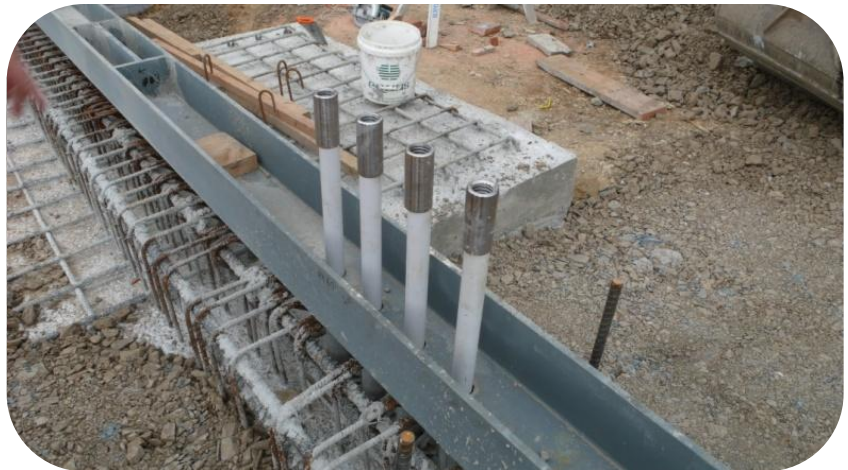
Figure E.5 Foundation for shear wall with steel shoe to seat shear wall and attachment points for Macalloy bars.
