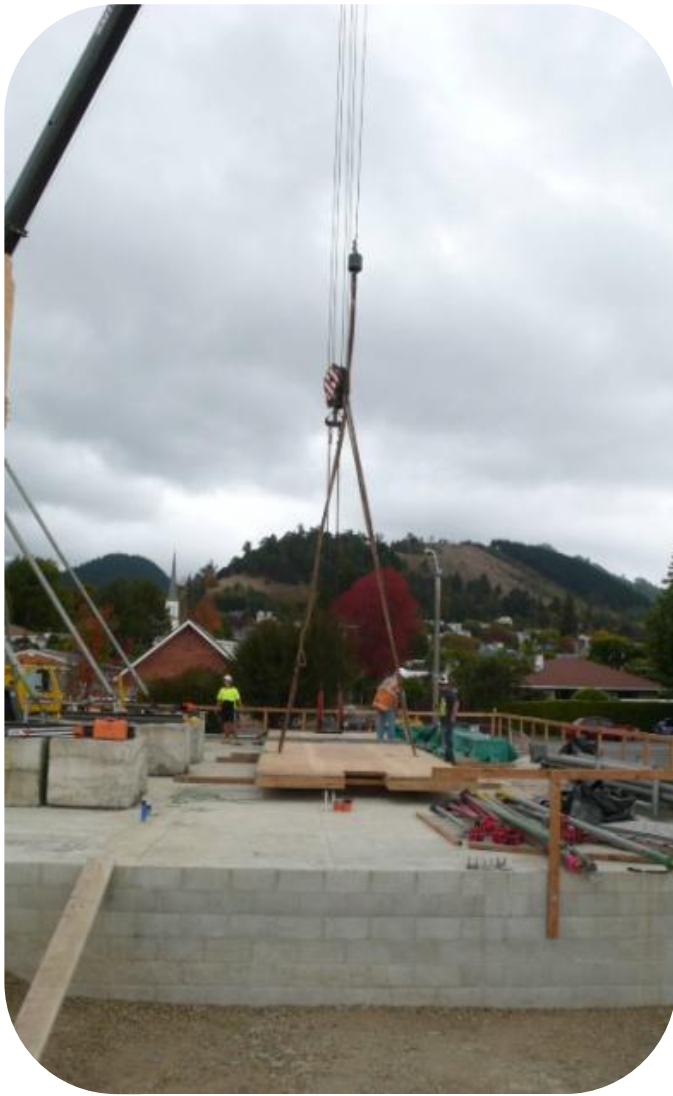
Figure E.10 Shear wall lifted from horizontal position into place. The walls are raised using two strops, tilted to vertical and lifted into place via the top strop.
