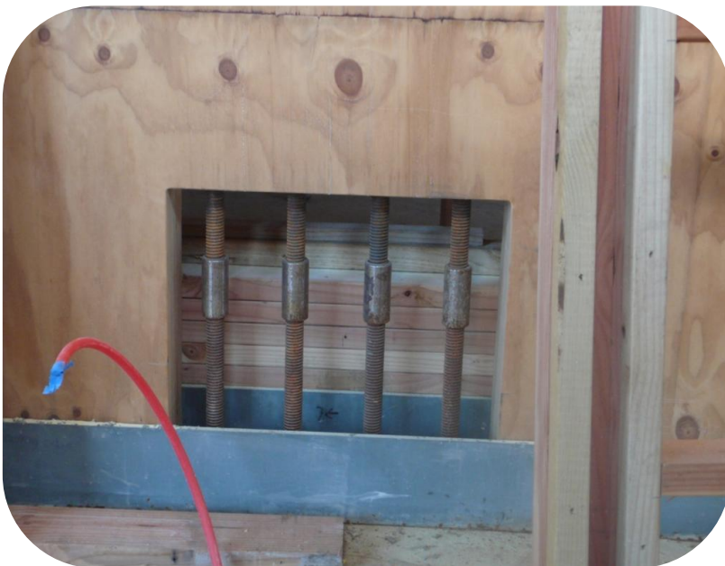
Figure E.19 Bottom of a shear wall showing the Macalloy bars attached into the anchoring points.
