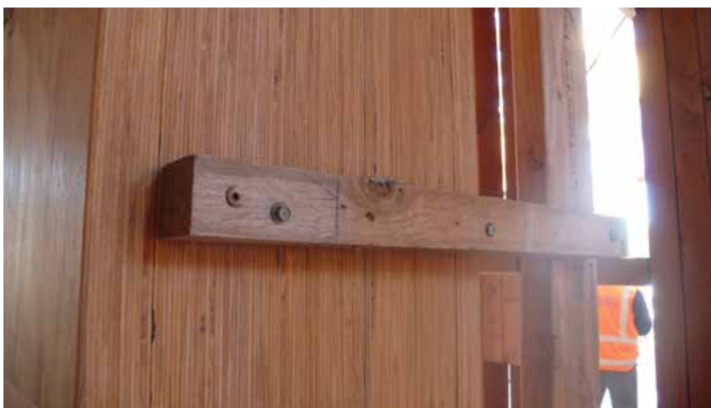
Figure 6.16: Attachment of temporary fixings to exposed structural elements, which damages the timber finish.
