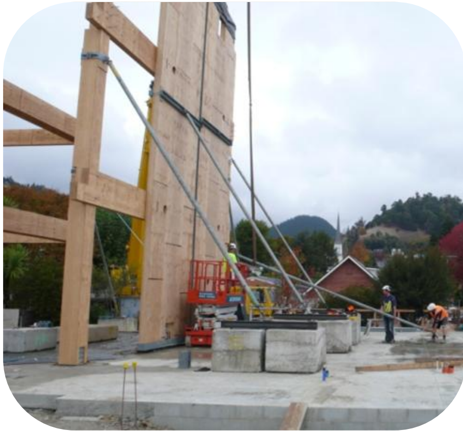
Figure E.15 Temporary bracing to right side of rear bay frame and shear walls. The temporary bracing stays in position until the floors have been constructed.
