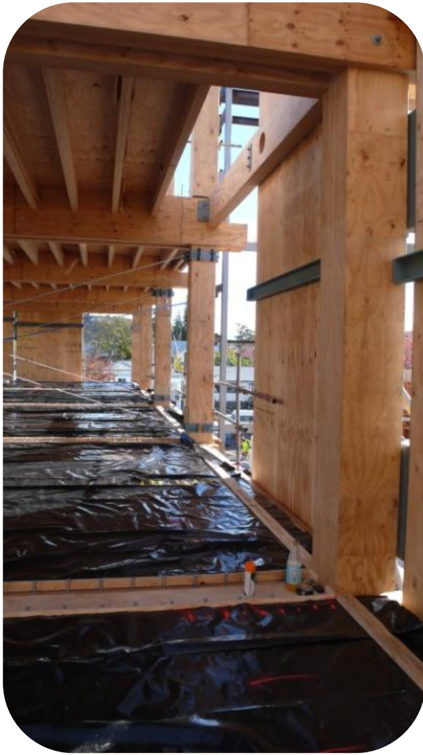
Figure E.24 Second floor level with plastic laid ready to pour concrete topping.
