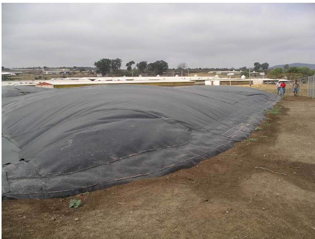
Figure 6-3: Covered anaerobic lagoon in Mexico.
