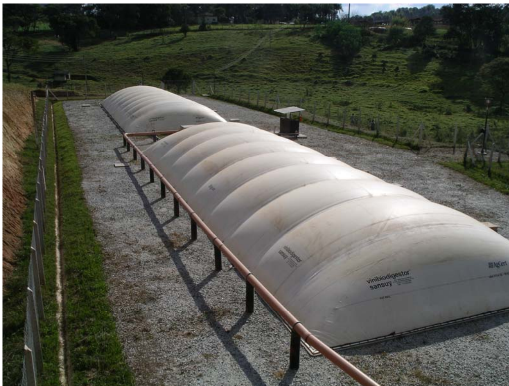
Figure 6-2: Covered anaerobic lagoon in Brazil
