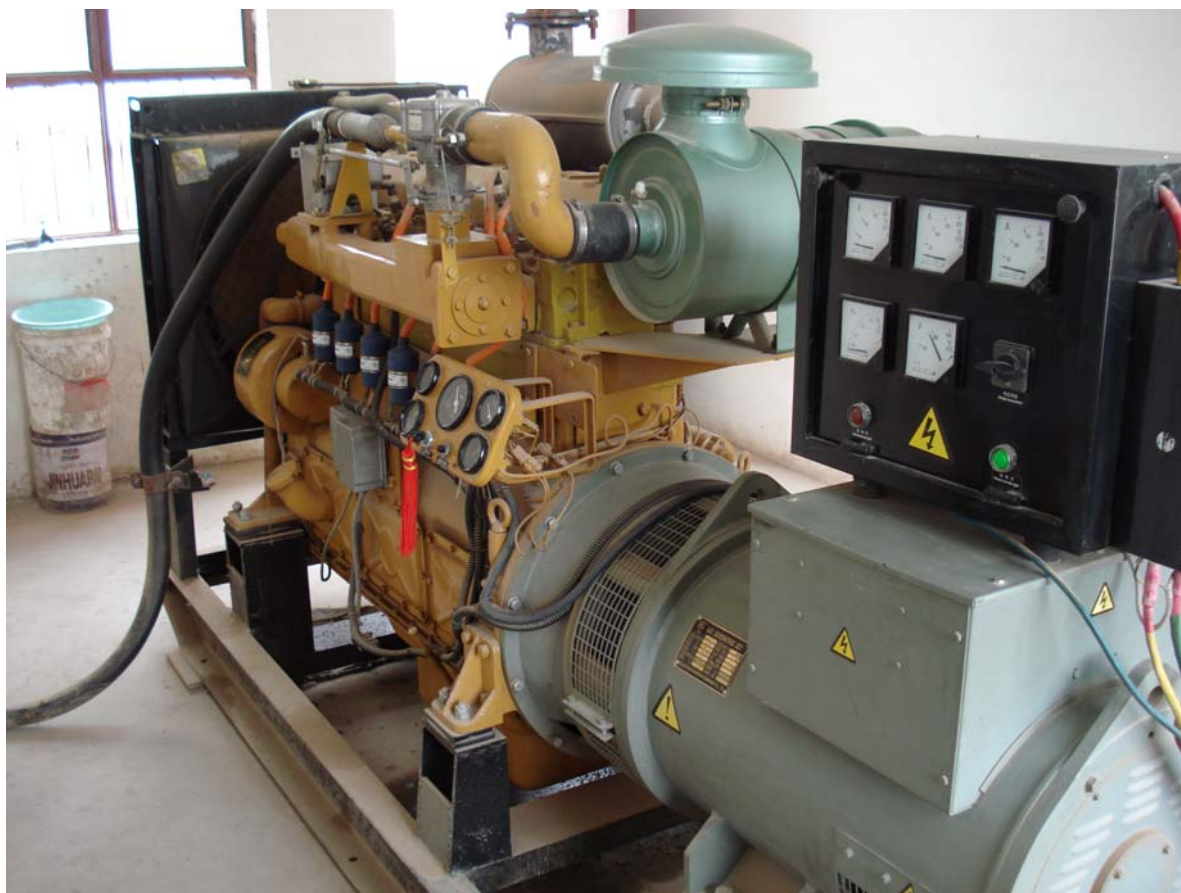
Figure 6-5: Biogas-diesel cogeneration engine for electricity generation
