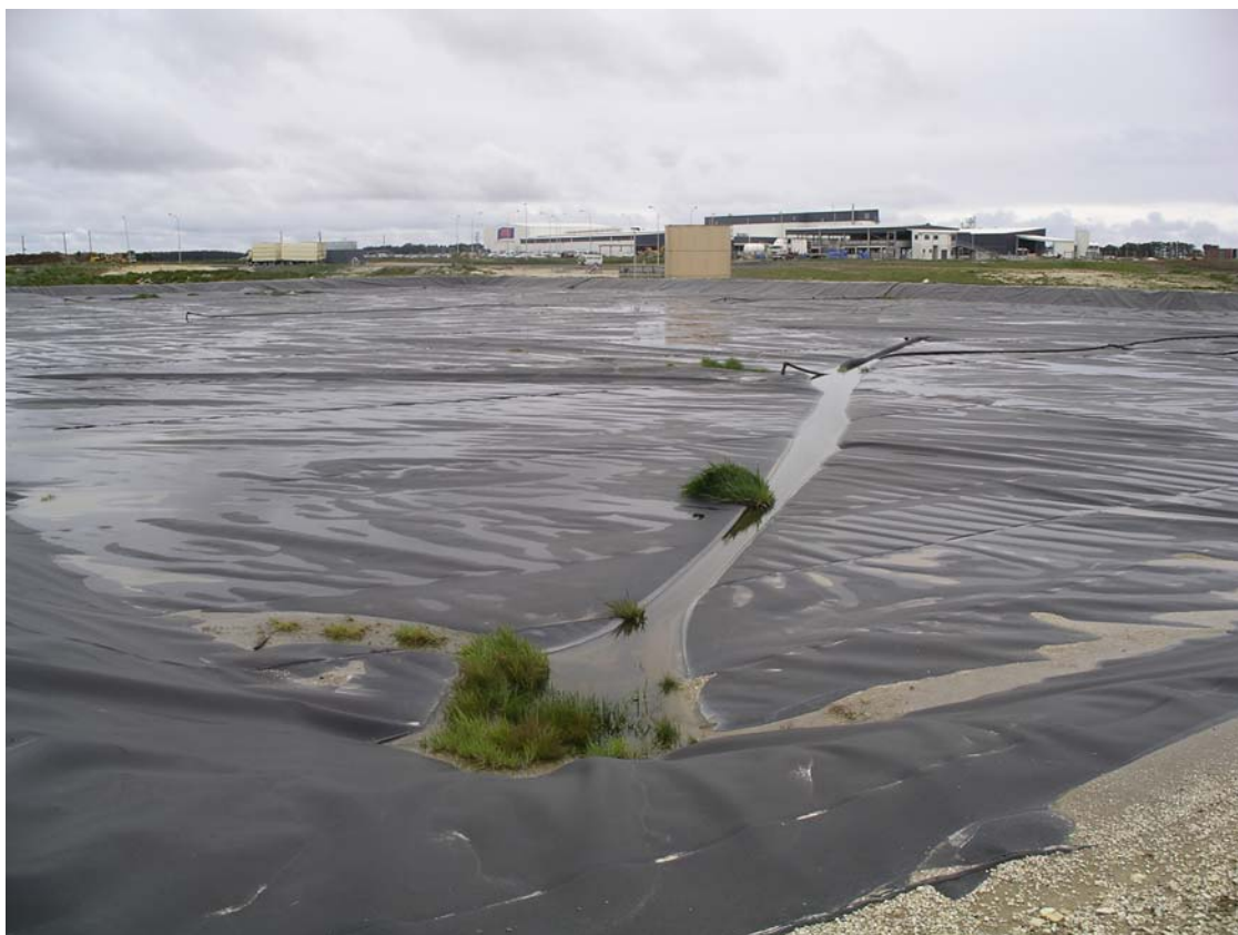
Figure 6-1: Covered anaerobic lagoon treating meat processing wastewater, Invercargill.
